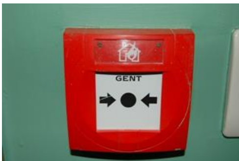
Fig 5. Gent Break Glass Unit.
