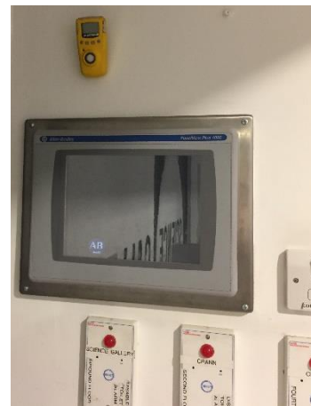
Figure 5 Gas Panel at CRANN
