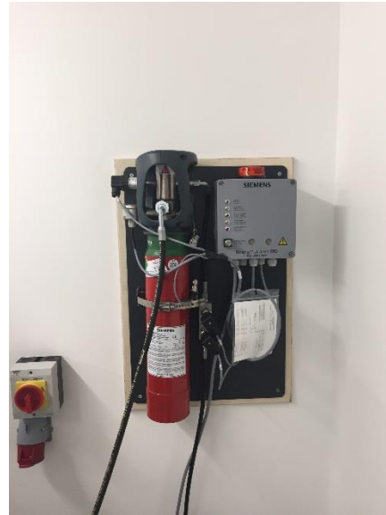
Fire suppression system for Realizer
