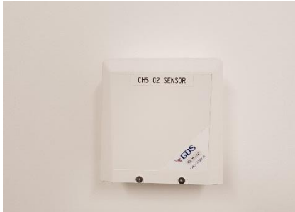
F Fig 3. Oxygen Depletion Sensor reception
