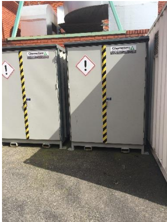
Metal outdoor shed for all metal powder storage
