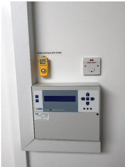
Alarm panel outside ARL main door
